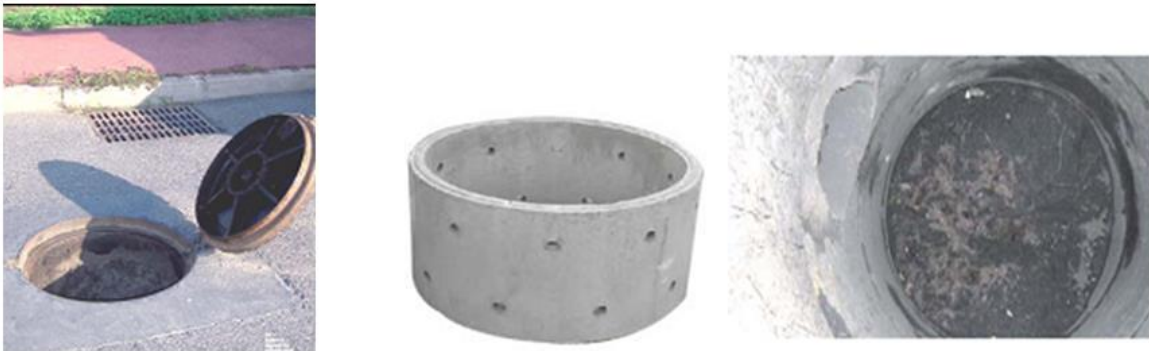
Fig. 2. Different views of infiltration wells, source: FIOGEP, 2010.
