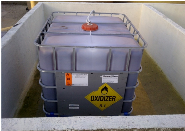
Figure 5. Type of container with sodium permanganate CARUSOL.
