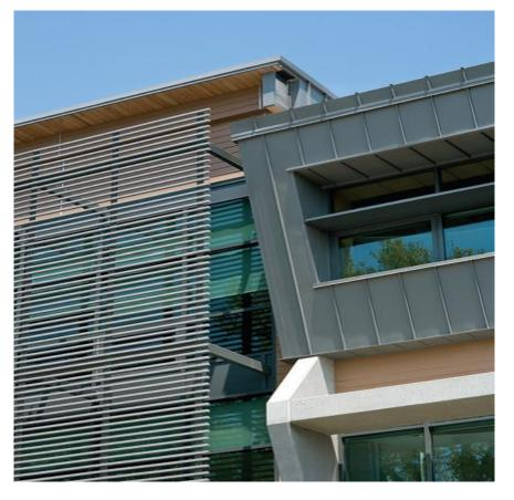
**Fig. 10.** Luis & Clark's office building, for the Missouri Ministry of Natural Resources, has been well integrated into solar control for glass envelope. (Source: BNIM)
